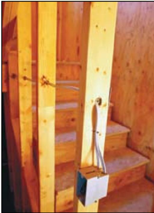
Nonmetallic sheathing helps protect wires from damage.
